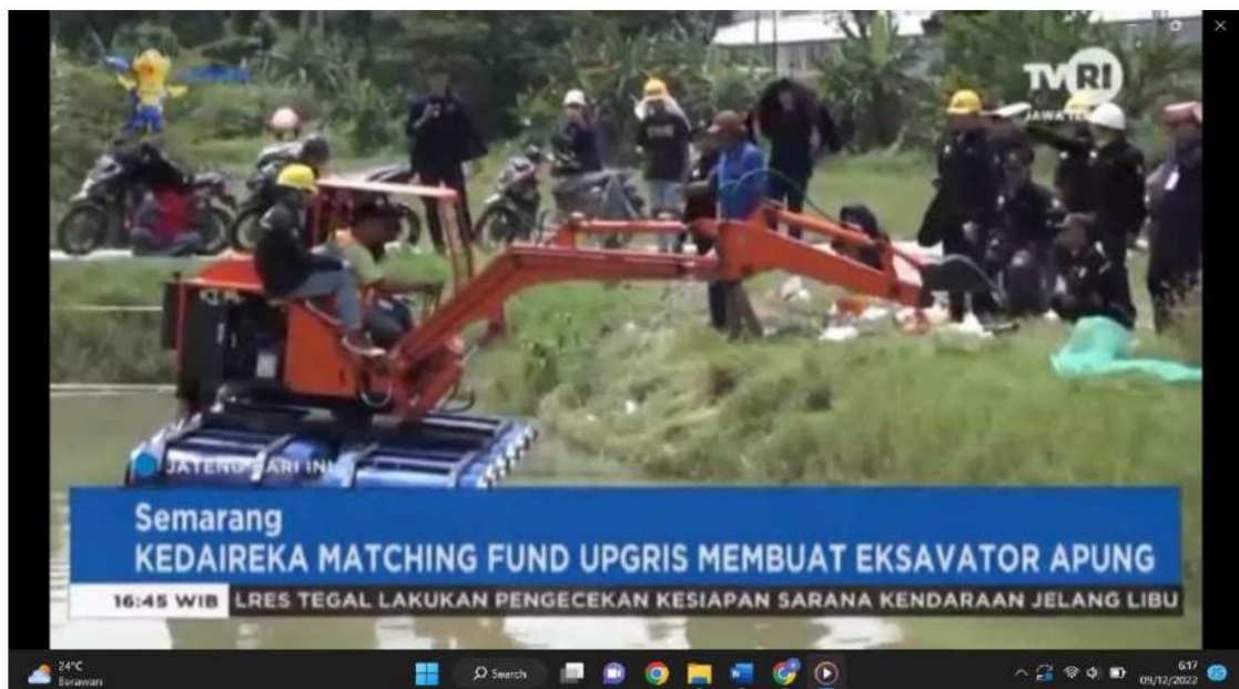
Figure 59 Trial of Floating Excavator Product in a pond Wijayakusuma Area, Semarang
